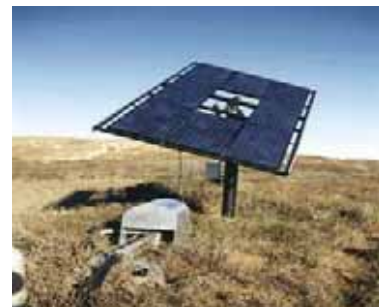
Solar Pumps Up to 5.8m 3 /h, 12 bar
