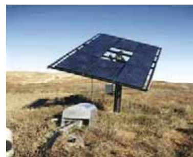
Solar Pumps Up to 5.8m 3 /h, 12 bar
