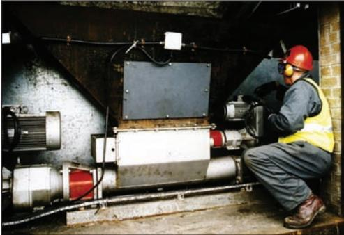
◀ A W064 model installed at a sewage treatment works to control sewage odours, caused by a belt press feeding dewatered sludge cake directly onto an open-air conveyor and into an open skip for disposal. The cast iron W064, with an integral bridge breaker fitted as an option, delivers the sludge cake at the required rate of 2.5m<sup>3</sup>/h and pressures of up to 12 bar. It operates eight hours per day, six days a week and daily fills up the four enclosed skips with sludge cake.
