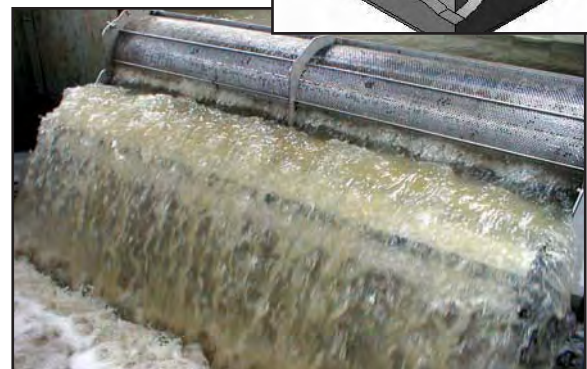
2 Stormscreens installed to screen storm overflows
