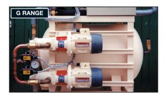
2 off CGG233R1/Y units on a 'domestic water module'. Duty approximately 2m³/h at 3 bar. This module distributes fresh water for domestic services such as toilets, showers, washbasins etc., on a tug currently based on the Solent. Built into the module is a calorifier for hot water service and U.V. treatment for potable (drinking) water.
