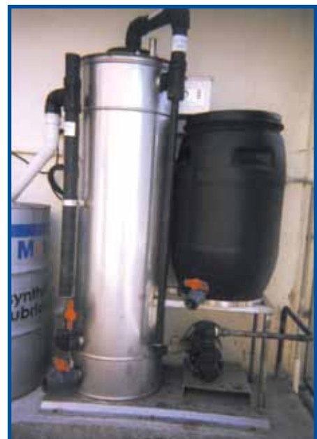
OILY WATER SEPARATOR
