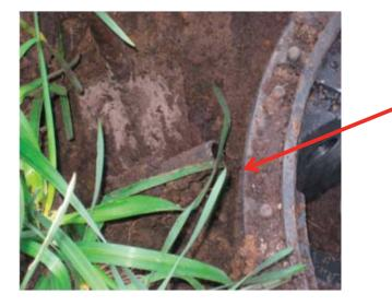
13. Remove rigid discharge line on the outside of the tank.
