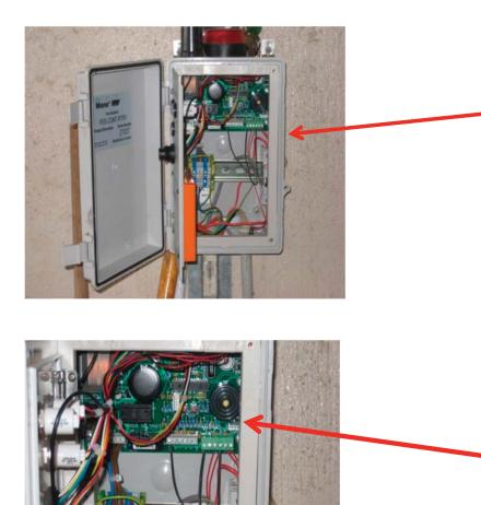
23. Change numbered wiring connection sequence in control box as per the IOM manual instructions/ diagram.
