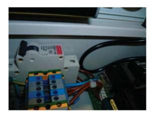
2. Turn off the circuit breaker for the pump.
