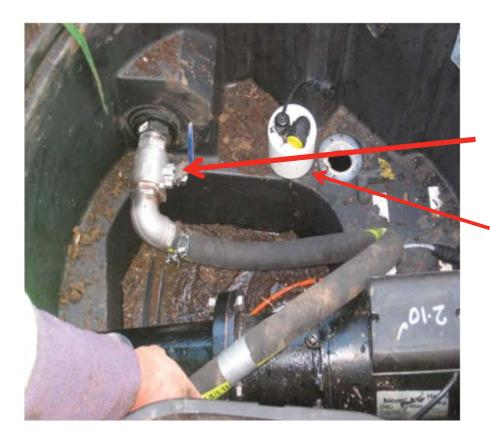
14. Install flexi discharge line as shown (existing gaskets and retaining nuts can be re-used)
