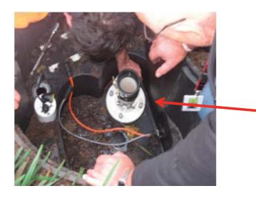
11. Install new telescopic pump inlet assembly.
