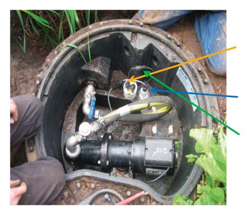
18. Remove existing level control cable plug and replace with the upgrade plug supplied. (refer to wiring diagram/ instructions in the IOM manual)
