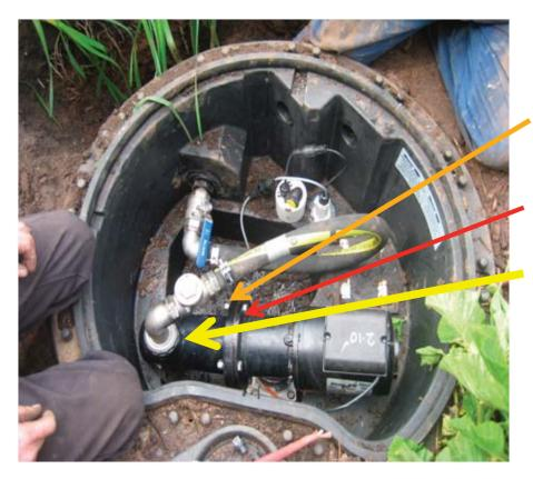
16. Remove the four bolts used to secure the pump discharge chamber to the pump inlet section.
